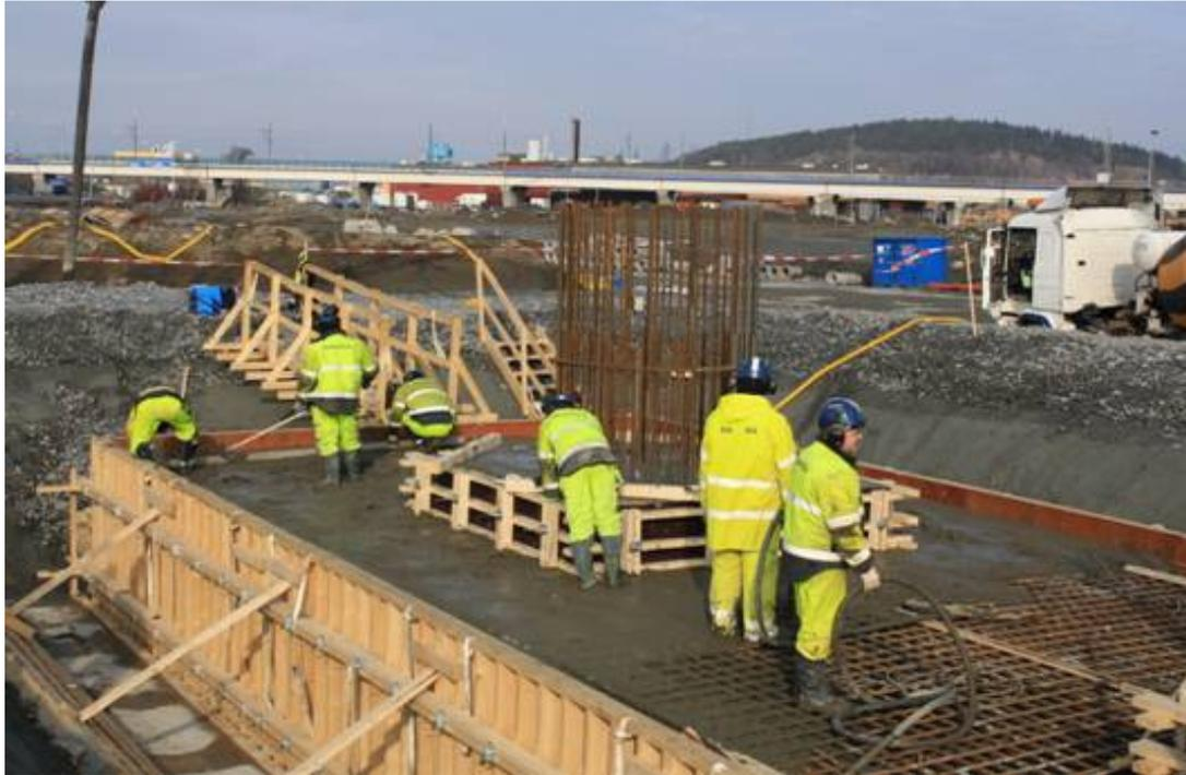
*Figure 1.4 Concrete is poured into the formwork*
