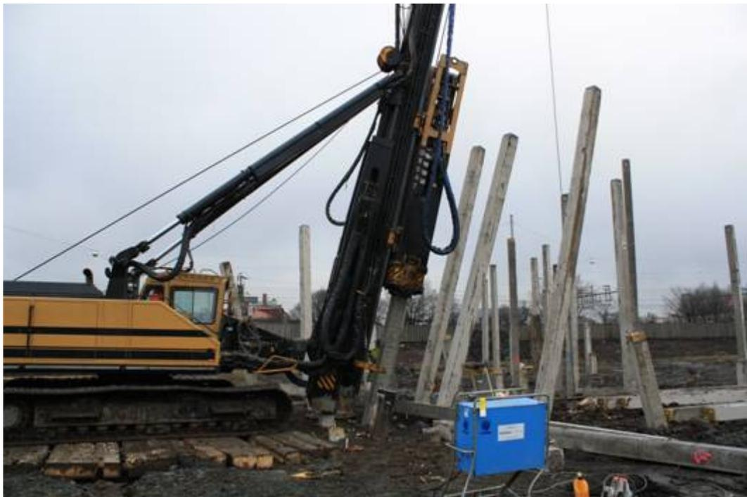
*Figure 1.1 Piles are driven into the ground*
