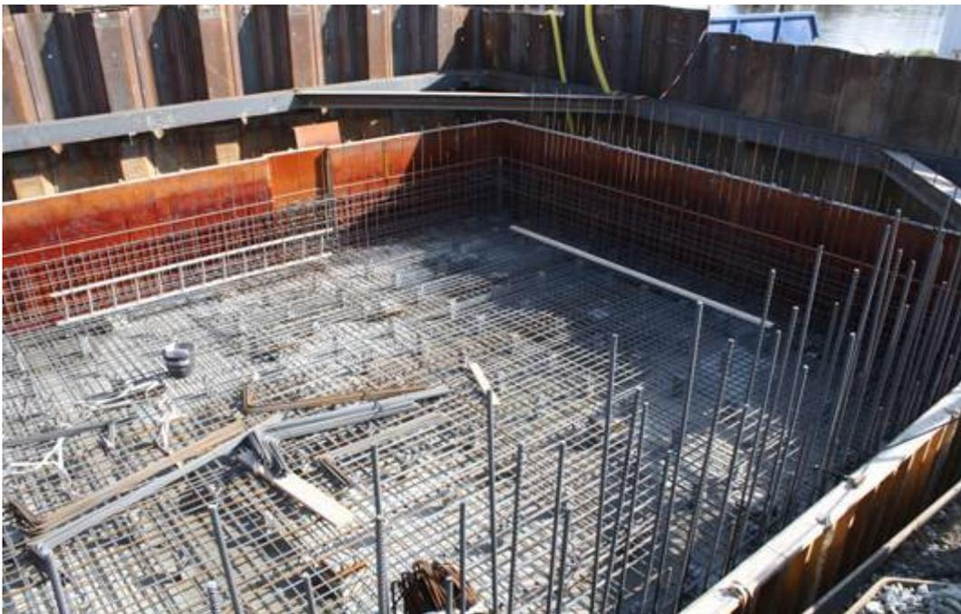
*Figure 1.3 Formwork and reinforcement of a pile cap*
