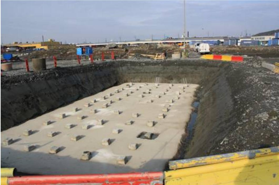
*Figure 1.2 Layer of blinding concrete cast over the piles*
