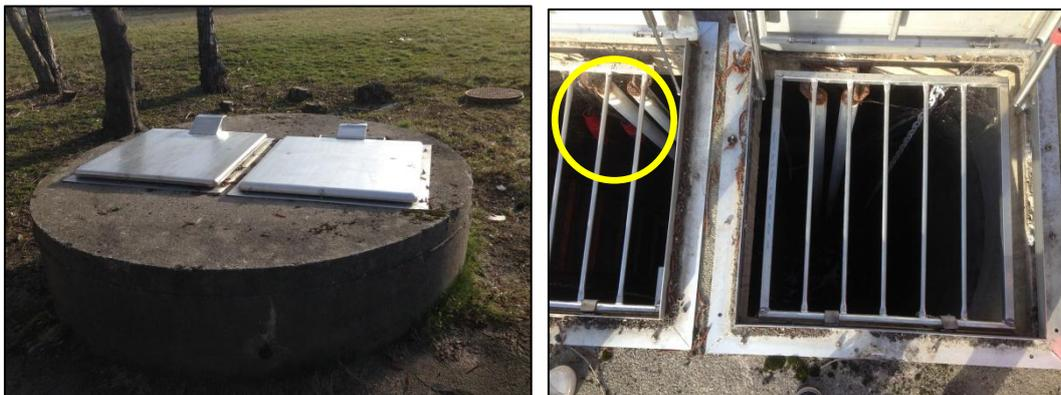
Figure 13 Example of a covered outdoor pumping chamber with submerged pumps. The power cord connections are marked with the yellow circle in the image to the right
