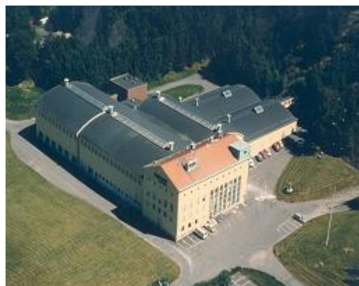
Picture 2: Alelyckan waterworks
