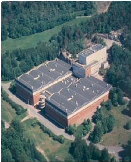
Picture 3: Lackarebäck waterworks
