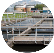
Picture 1: Water Treatment Plant
