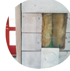
Picture 42: Trust Windows Ekopark Strömstad a
