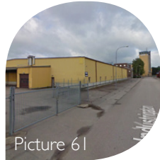
SANDEN- INDUSTRIAL SHED
