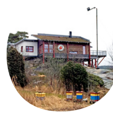
Picture 40: Exterior Ekopark Strömstad a
