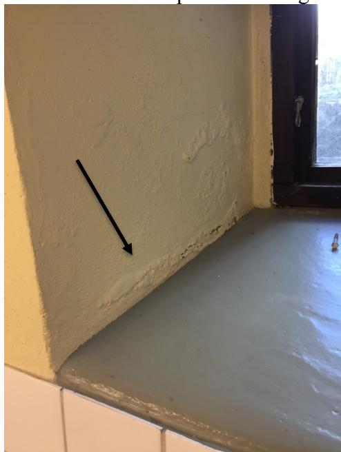
Figure 5.15 Flaking paint on foundation wall.
