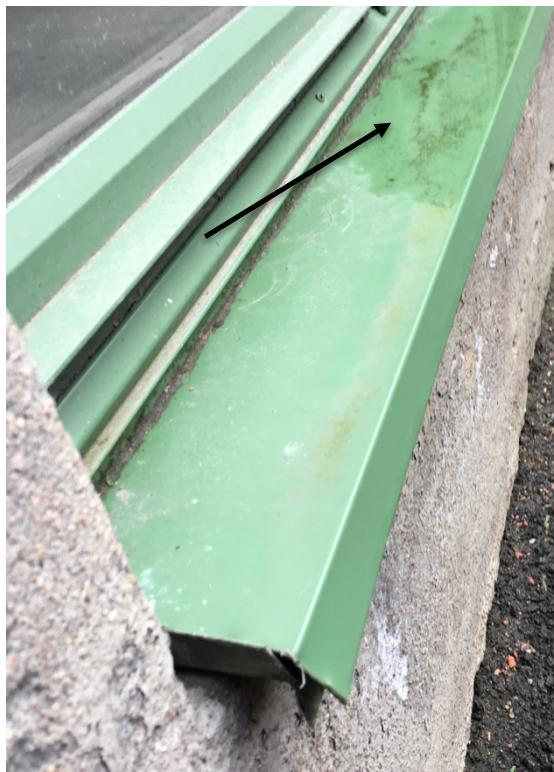
Figure 5.10 Difference in inclination of window ledges resulting in standing water.
