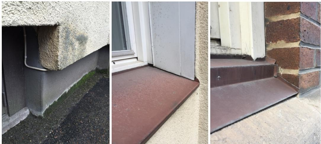
*Figure 5.4 Left: Added insulation on the wall facing the yard. Middle: Window and wall connection facing the yard. Right: Window and wall connection facing the street.*
