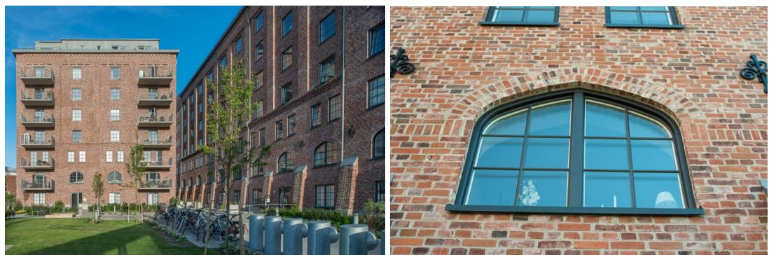
*Figure 4.4 Example of a new sandwich element with remounted bricks. Photos: Strängbetong (2016).*
