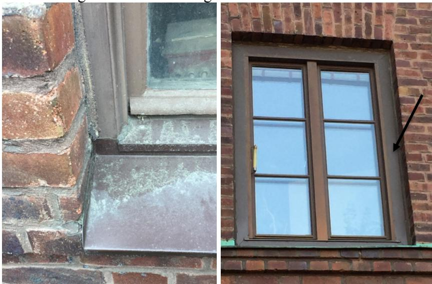
Figure 5.17 Left: Original wooden window. Right: Frame-in-frame window.
