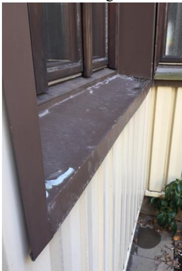
Figure 5.14 Changed window and its connection to the corrugated steel.
