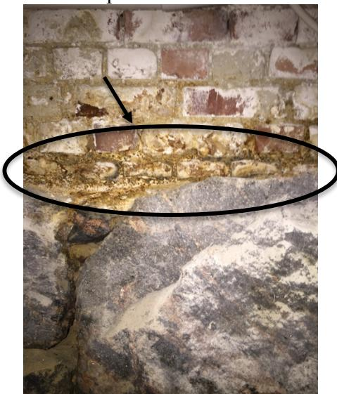
*Figure 5.5 Design and construction of the foundation wall with discolorations.*
