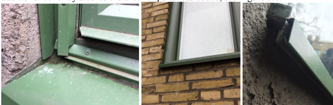
Figure 5.8 Left: Added cover to a window in the basement wall. The wooden frame is visible beneath the cover plates. Middle: Added cover to a window of an apartment. The wooden frame was less visible than in the previous figure. Right: New and old window ledge.
