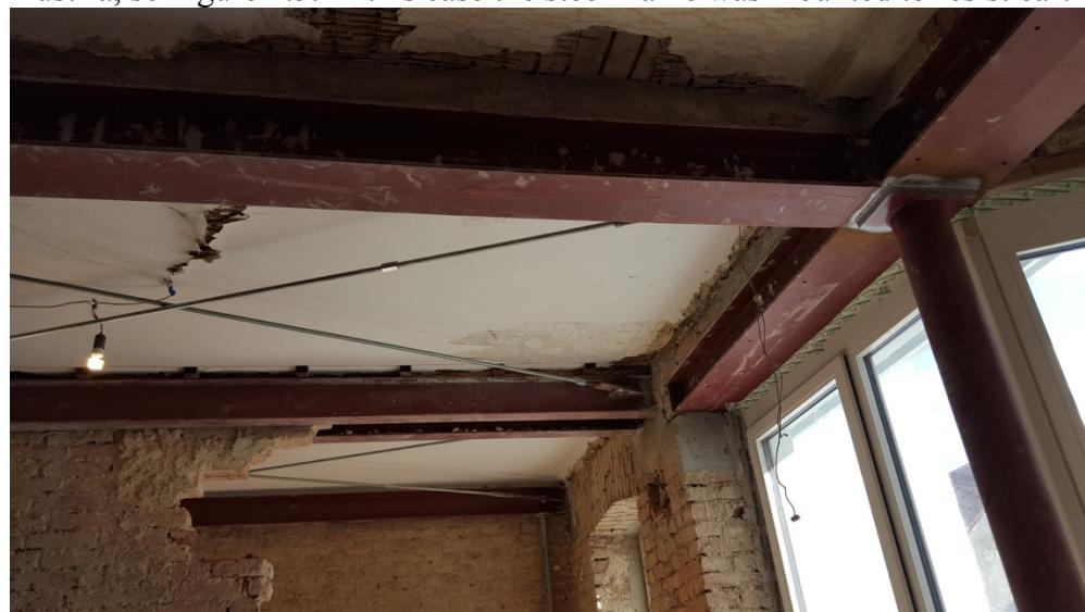
Figure 4.5 New steel frame in an old brick building in Vienna. Photo: Pär Johansson.
