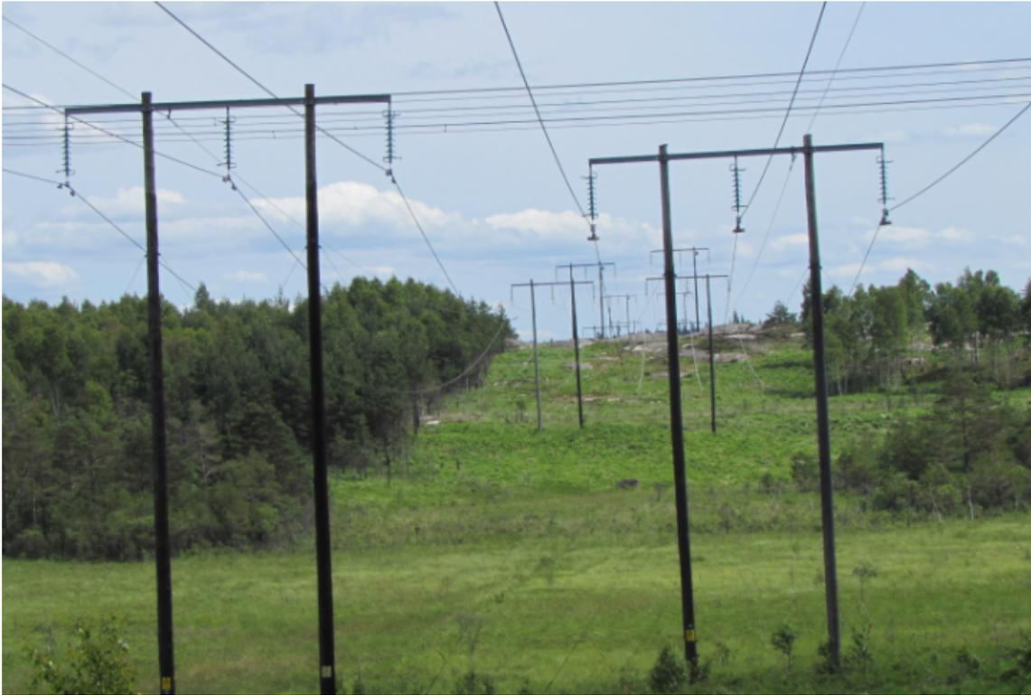
**Figure 3.4:** Wood portal tower with one shield wire and insulator strings with arcing horns.
