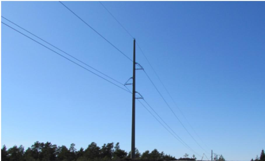
**Figure 3.8:** Concrete tower with a vertical phase displacement and one shield wire.
