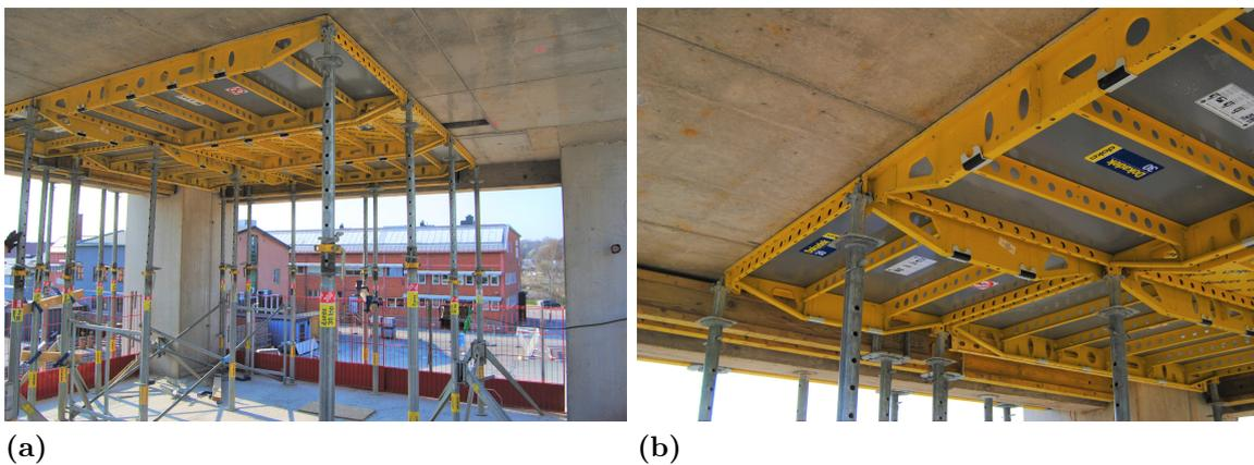
**Figure 2.10:** *Example of a soffit formwork supported by props.*
