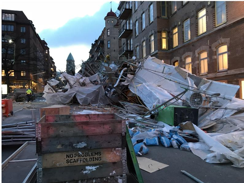
**Figure 4.5:** *The collapse of the façade scaffolding along Engelbrektskatan in Gothenburg (Hjelmgren, 2018).*
