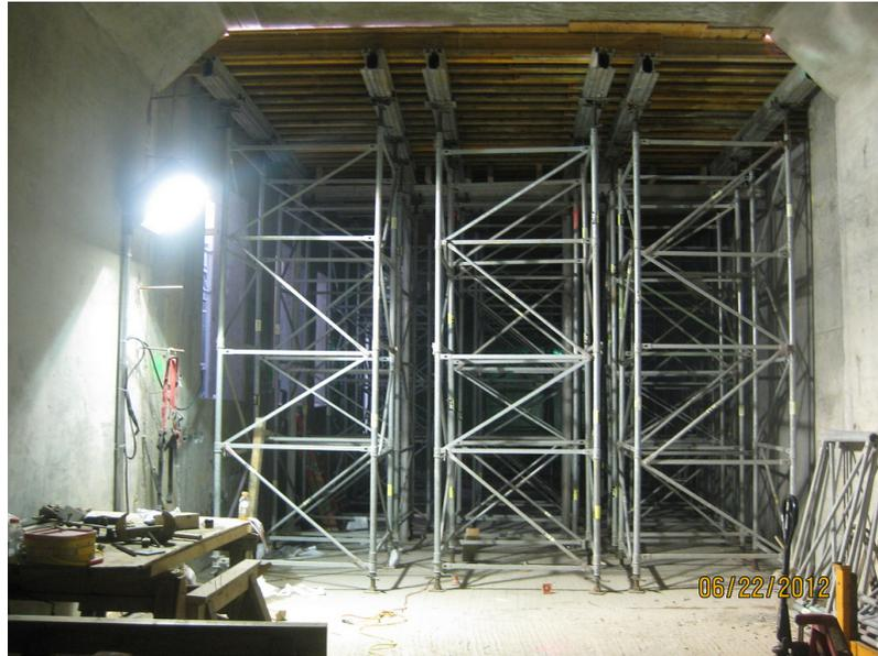
**Figure 2.2:** *Falsework supporting the soffit formwork where the permanent concrete structure is cast (MTA Capital Construction Mega Projects, 2012).*
