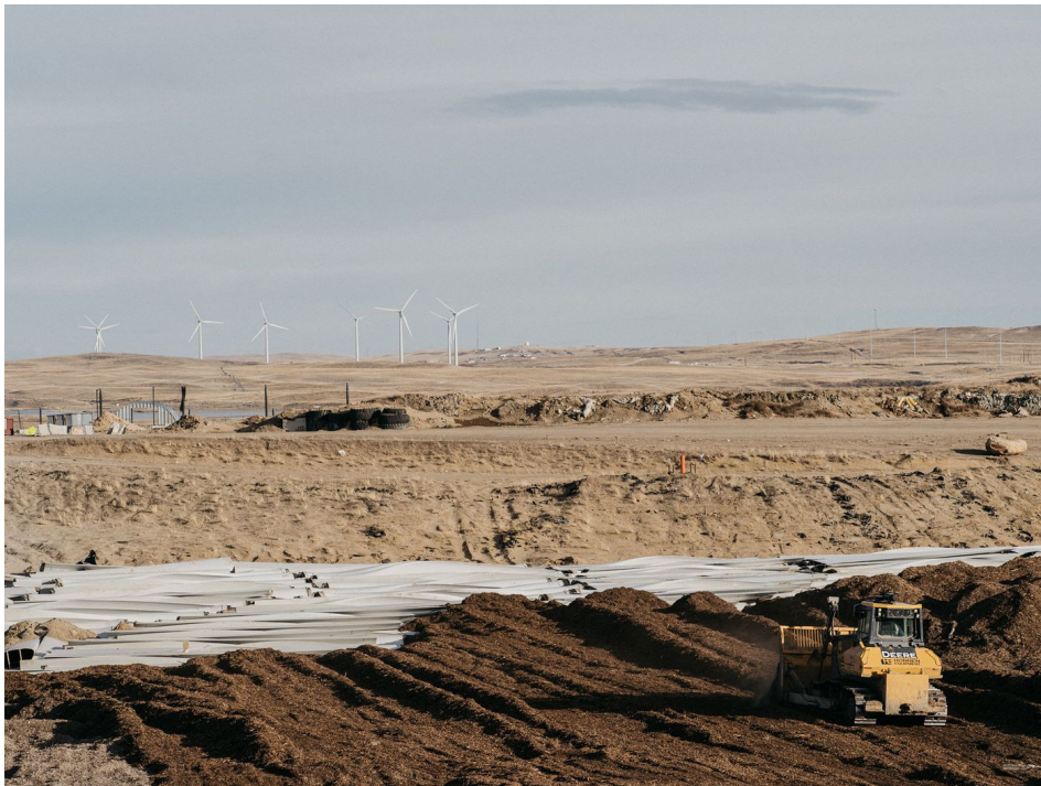
Figure 2.8: Wind turbine blades being buried at Casper Regional Landfill. Photographer: Benjamin Rasmussen for Bloomberg Green (C. Martin, 2020).
