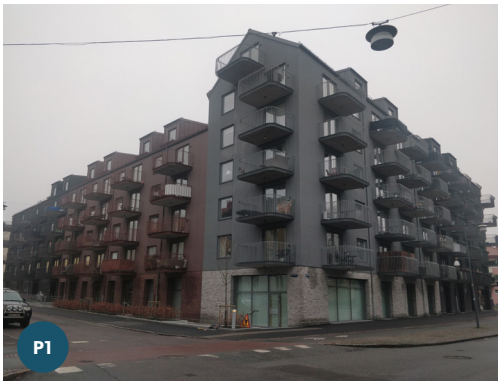
Figure 6.28 New residential building
