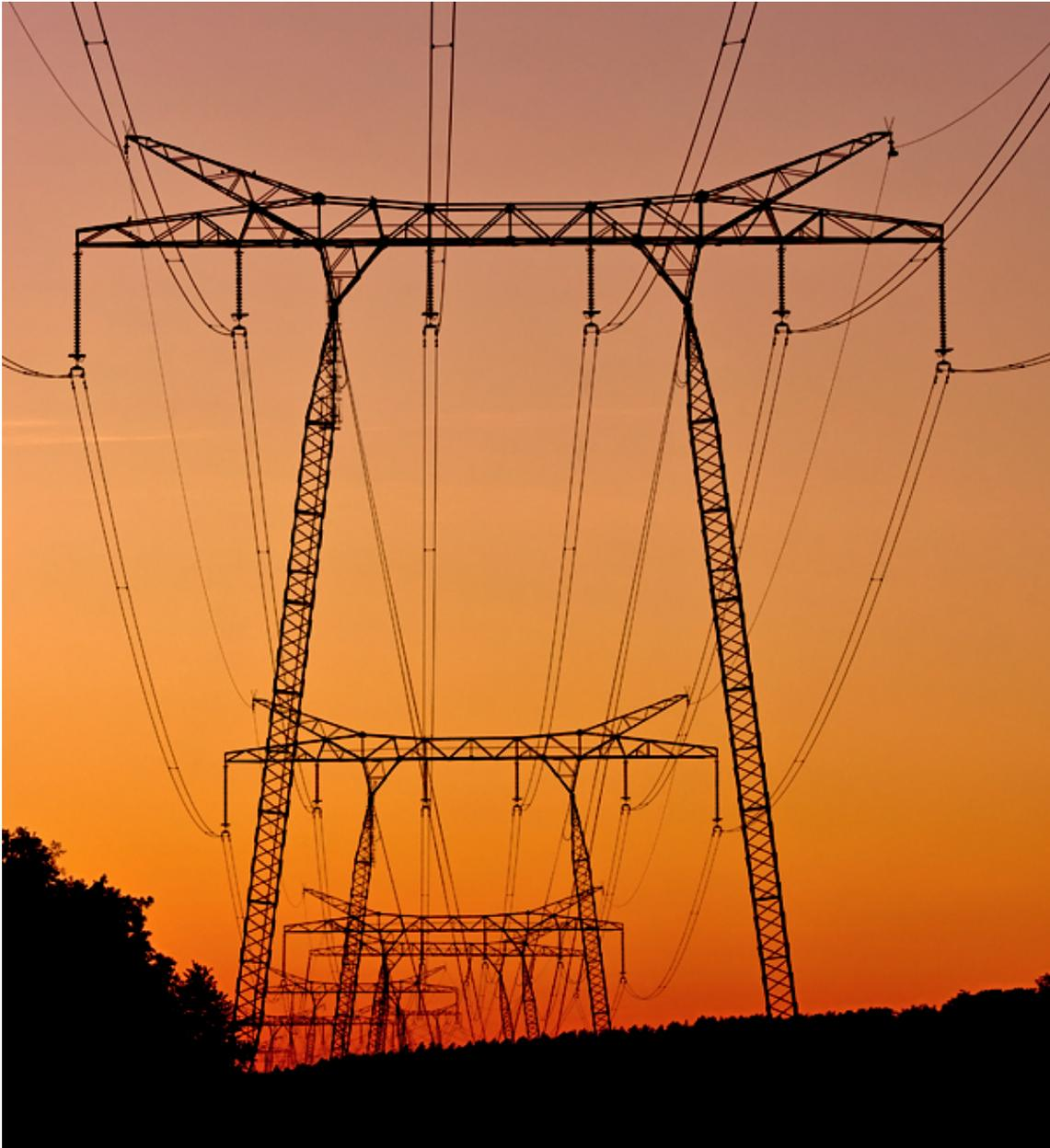
**Figure 2.5:** Increased insulation level on the outer phases due to large shielding angles at a tower used in the Swedish grid which was originally intended to be used for a 800 kV line but is instead used for two 400 kV lines. Photo taken by Puggen.
