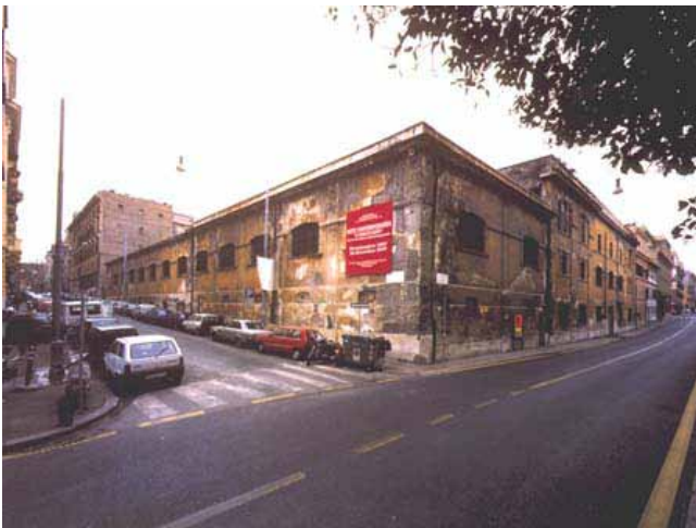
1. View of the corner of Via Nizza and Via Cagliari (photo from the competition program)
