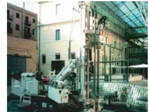
Investigations of the ground
