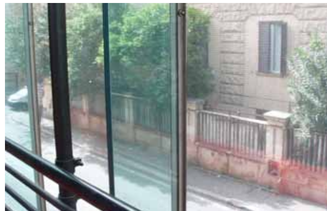
The steel mesh seen in a window
