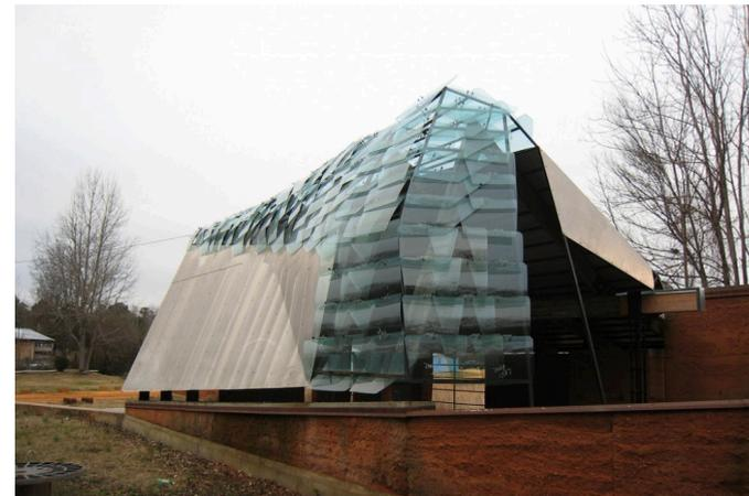
Fig. 23. The Manson Bend Glass Chapel by Rural studio with layered glass facade made of thrown away car windscreens. The shape of Rural Studios project usually grow from experiments with materials at hand.
