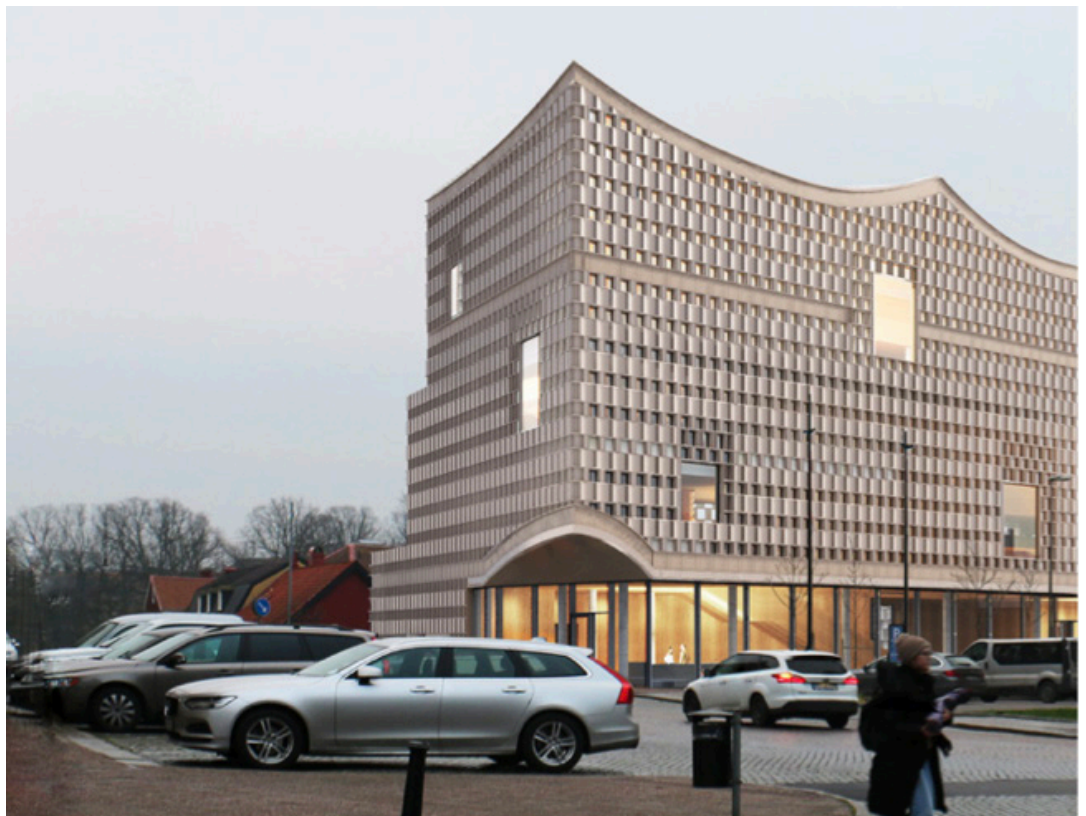
(Fig. X) Last variation of new culture house, Dorte Mandrup, Visualization by MIR
