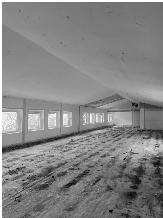
Current state of upper floor
