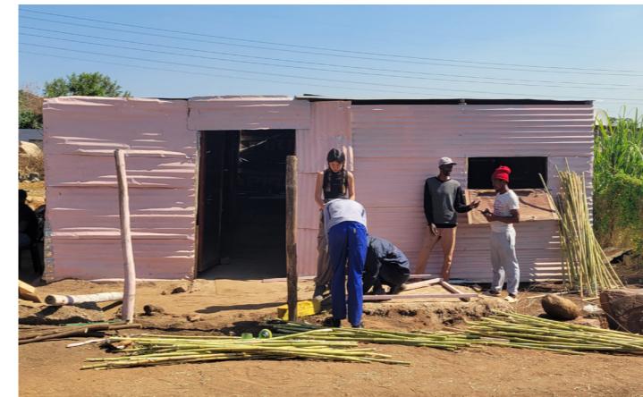
Replacing the old fence with a new
