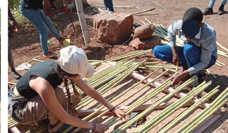
Construction of new gate and fence.
