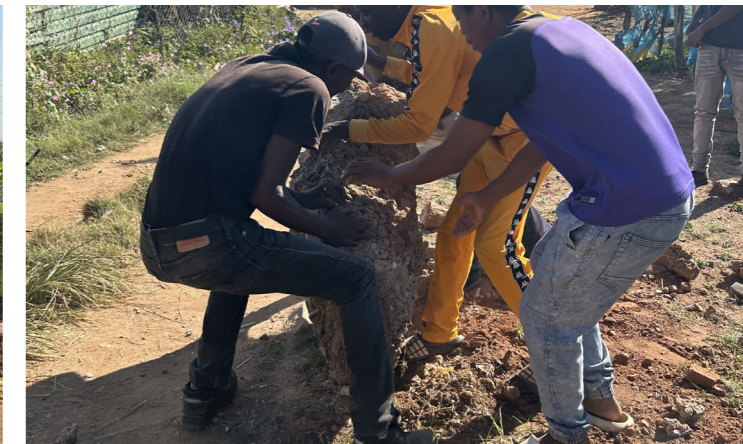
Clearing space on the road
