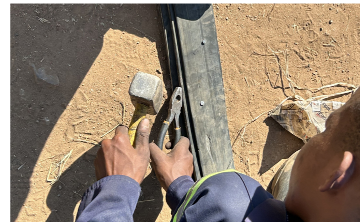
Building a speedbump to slow down traffic.
