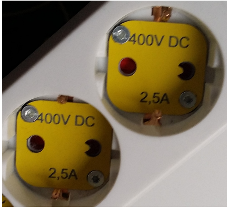
Figure 3.1: Specially made socket outlet for DC, picture is taken at the Swedish Department of Energy Headquarters in Eskilstuna.
