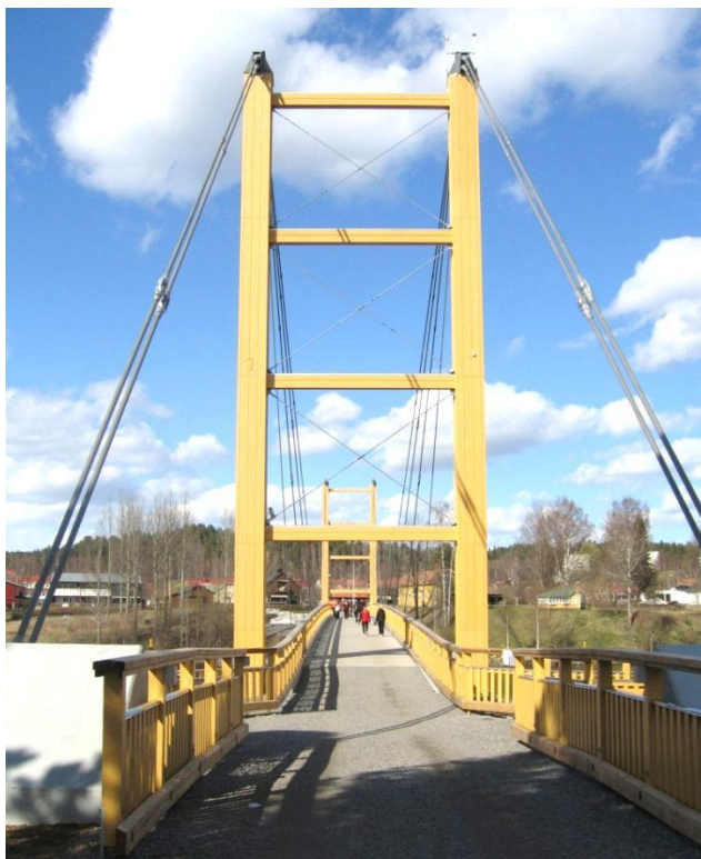
Figure 11 The south pylon of Älvsbackabron with its anchorage cables and concrete foundations
