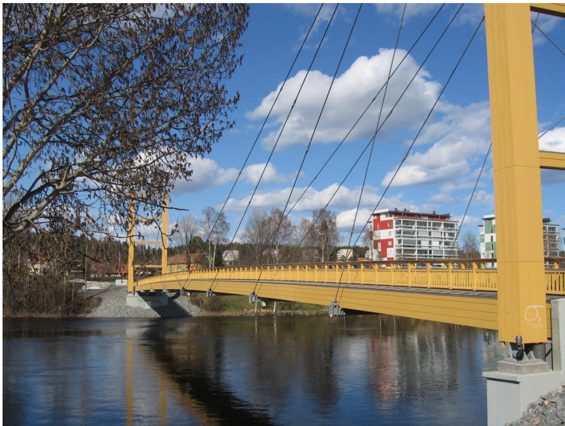
Figure 9 The slender profile of Älvsbackabron. The picture is taken from Anderstorp located on the south side of the river.
