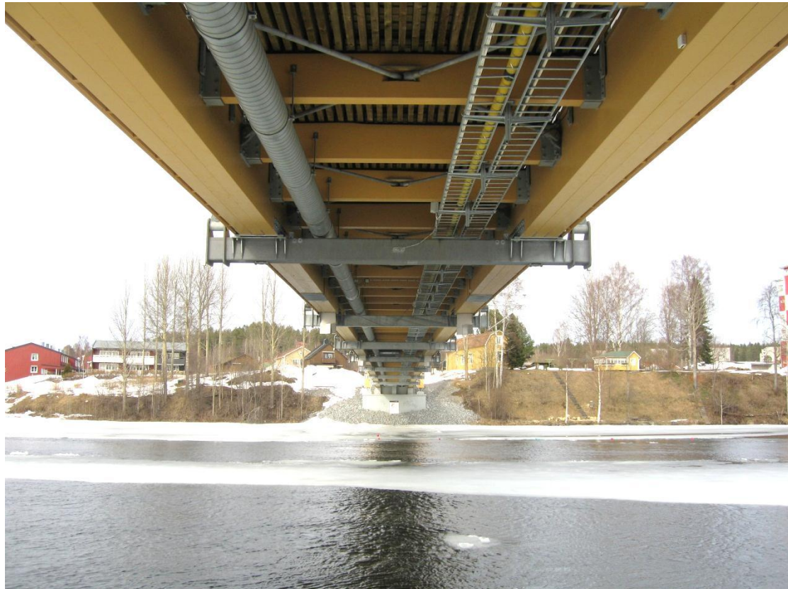
Figure 12 Älvsbackabron from below. The main beams are supported by steel cross beams to which the cables are attached. The glulam cross beams, timber purlins and steel cross bracing can also be seen.
