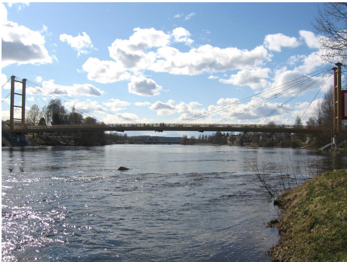
Figure 14 The scenic view of Älvsbackabron. The new bridge is supposed to improve the living standard for the people of Skellefteå.
