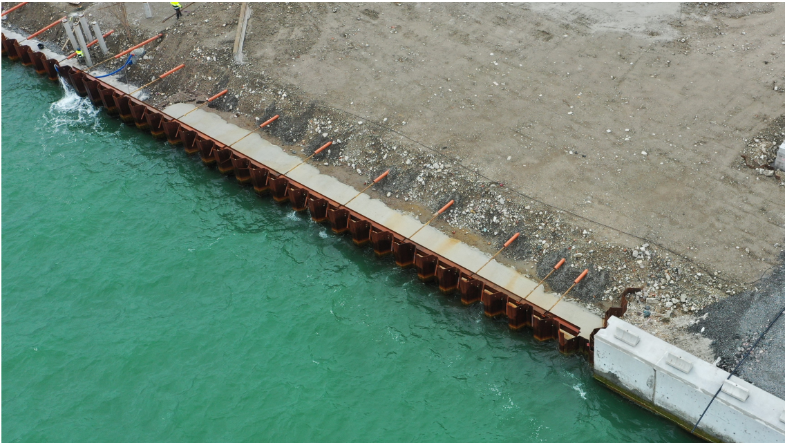
Figure 3.3: Installed sheet piles, before installation of the capping beam (PEAB, 2021).
