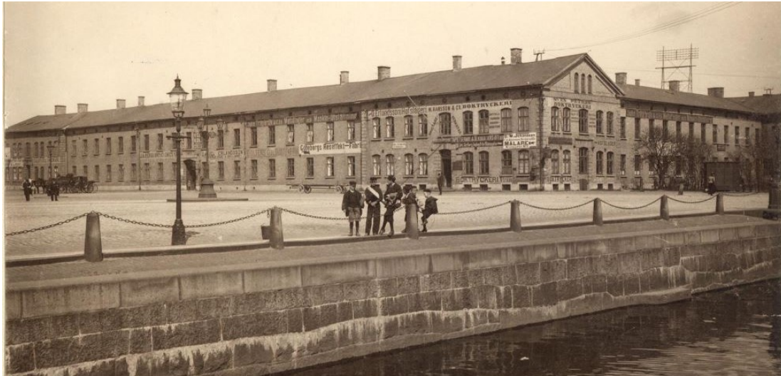
Figure 2.2: An example of a gravitational retaining wall found in Gothenburg, Sweden close to the Centralstation taken around 1900 (Vårt Göteborg, Göteborgs stads tidning, 2023).
