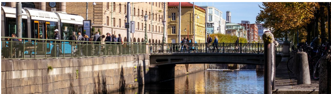
Figure 2.3: The quay wall around the central station as it looks in 2025 (Göteborg stad, 2025).
