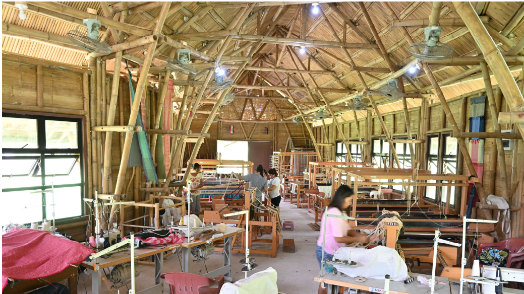
Figure 9 Inside view of the case-study building: Kanya Kawayan weaving centre in Nasugbu, Philippines.
