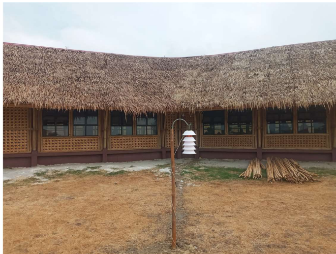
Figure 17 Outdoor measuring equipment in the case-study building. Technical details in Appendix B.
