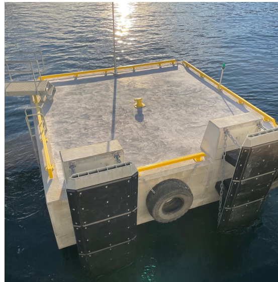
Figure 1.2: Modern mooring dolphin featuring concrete pile cap. Comment: Adapted from: Dykdalber Flekkefjord 005 Vest Betong [photo], of Vest Betong, 2021, Vestbetong.no/prosjekt/dykdalber-flekkefjord/. Reprinted with permission.
