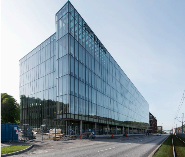
Figure 3.9 Image of K21 building in Mölndal (57°40'09.4"N 12°00'37.3"E). On one side a double-skin façade, on the other side an ordinary glazed façade. Retrieved June 13 th , 2019 from http://www.acc-glas.se/projekt/krokslatts-fabriker-k21/ .
