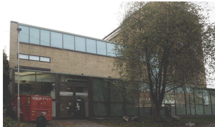
Gothenburg Museum of Art - East Etagera - 4 Falkhallen - 5
