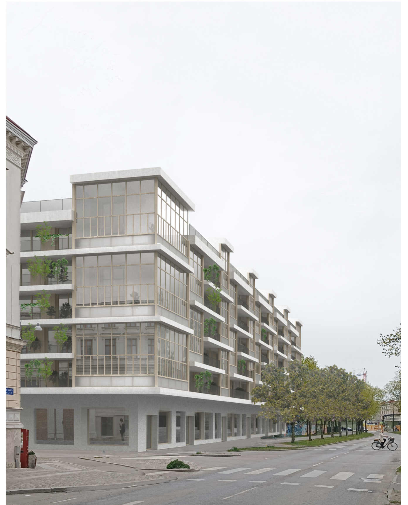
Exterior - south-west facade
