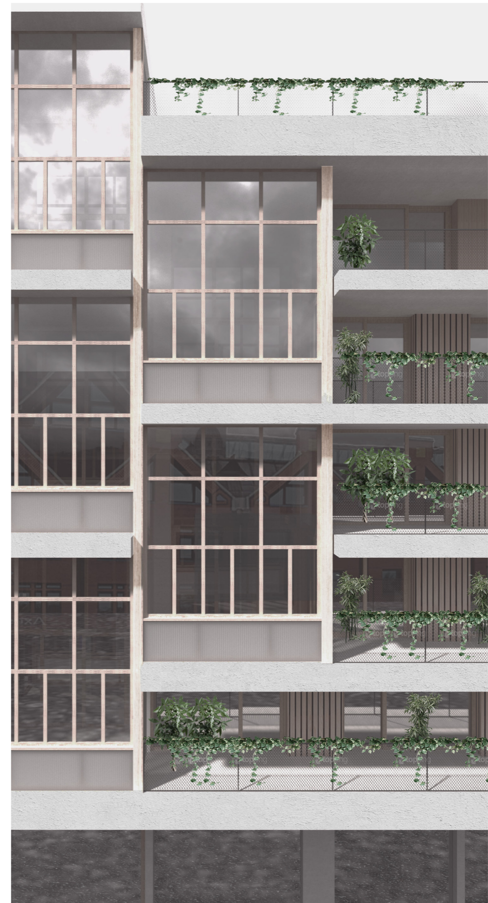
Exterior - southern facade
