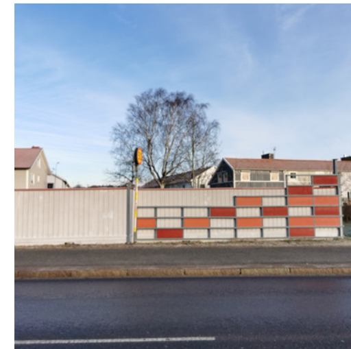
Walls to protect the neighborhood from noise
