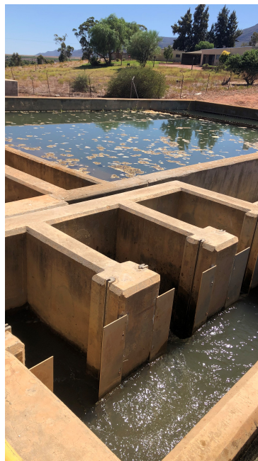
Figure 3.3: Horizontal sedimentation at Piketberg DWTP.
