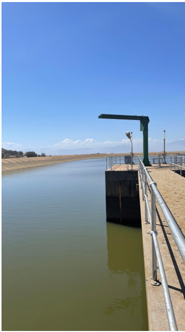
Figure 3.6: Raw water storage at Withoogte DWTP.
