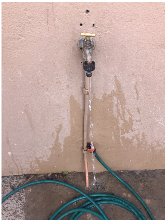
Figure 3.15: Sampling of drinking water at Piketberg DWTP.
