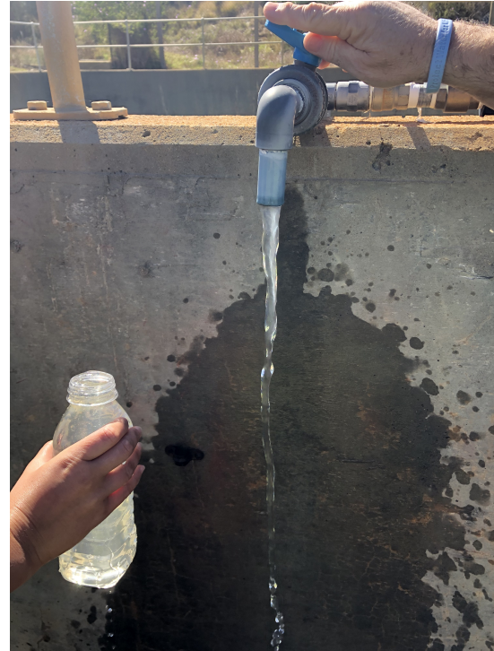
Figure 3.14: Sampling of raw water at Withoogte DWTP.
