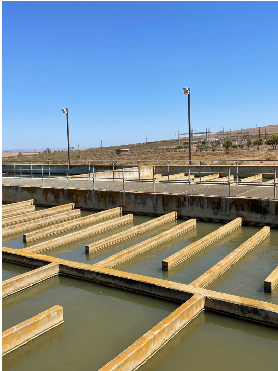
Figure 3.9: Horizontal sedimentation at Withoogte DWTP.
