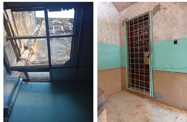
Fig67. The existing metal roof. View from groundfloor
