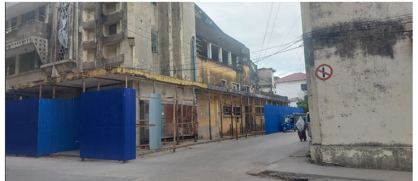
Fig.15 Majestic Cinema scaffolding
