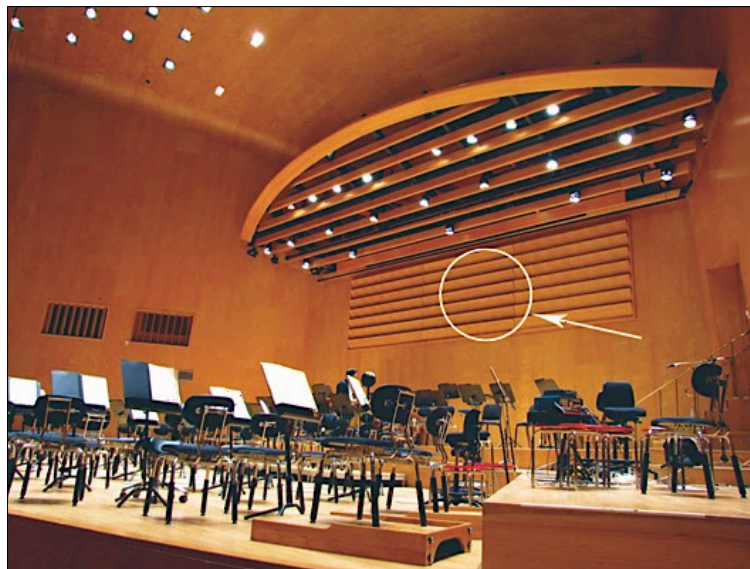
Figure 6.1. The concert hall of the Göteborgs Konserthus (Sweden) with variable acoustic conditions 1 (wall reflectors were open) (Photo by Maryam Sadeghi)
