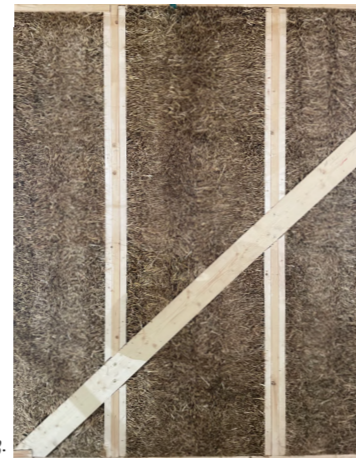
Image 1. The barn - "factory" Image 2. Pressed straw bale Image 3. Section of prefab panels
