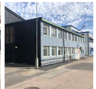
The small office building
