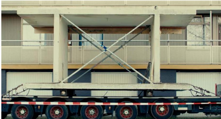
Figure 25. Extracted 3D units from the Super Circular Estate project in the Netherlands (Elma Durmisevic, 2019).
