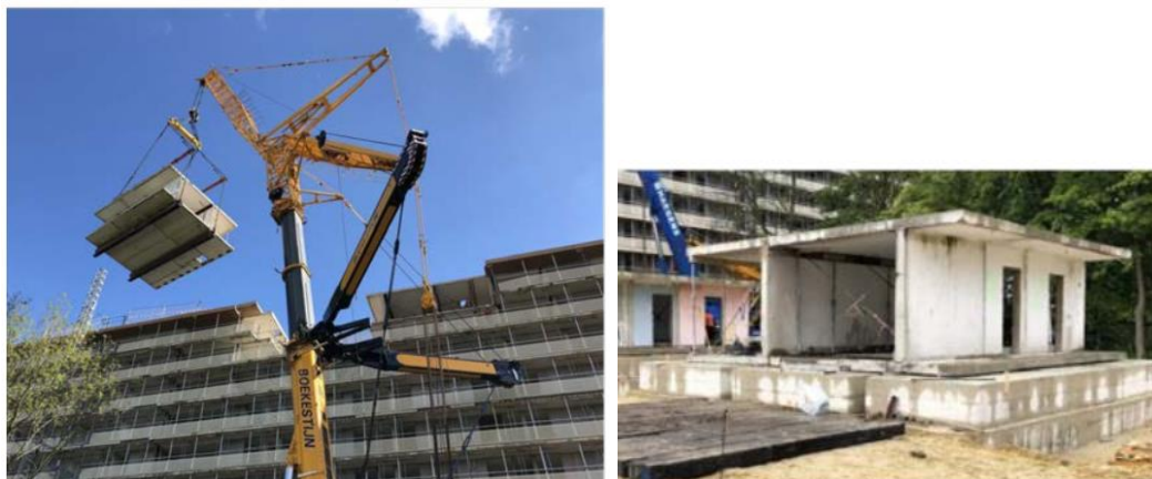
Figure 26. Lifting out and reinstallation of the 3D units (Elma Durmisevic, 2019).
