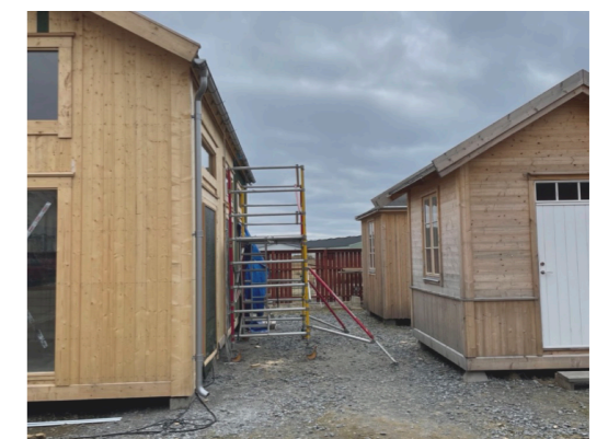
Figure 18. Ongoing projects in the building area at Egnahemsfabriken.
