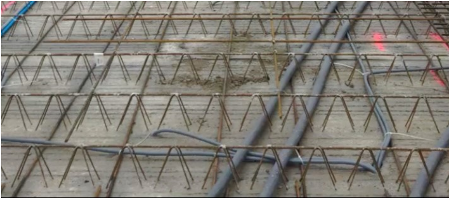
Figure 3.3: Filigree elements mounted at construction site.
