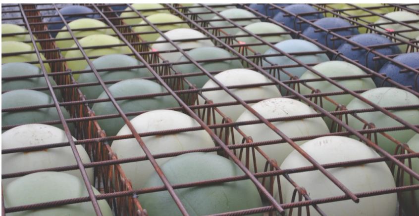
Figure 5.2: Voided biaxial slab (Mortensen, 2016).
