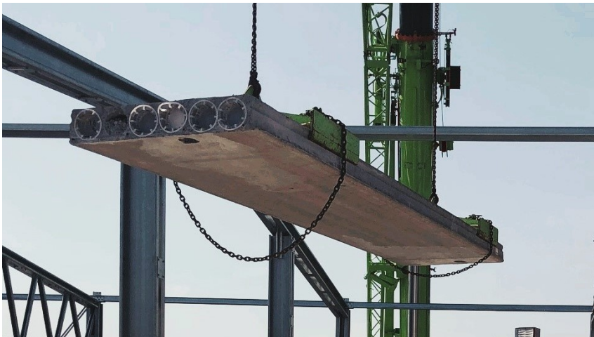
Figure 3.1: Hollow core element (type HD/f-200) mounted by crane at construction site.
