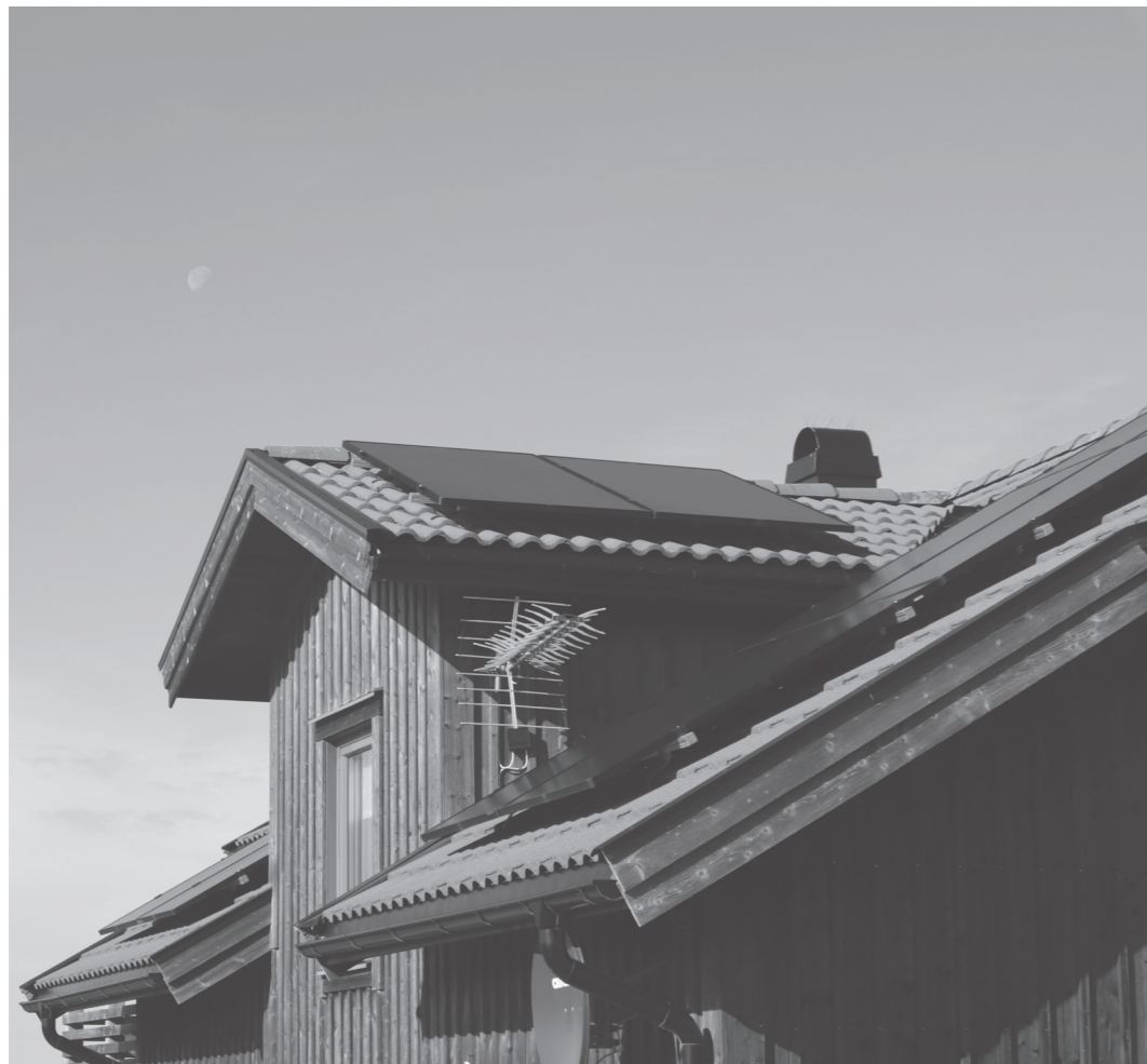
Photo 3. Solarpanels on existing roof in Ulebergshamn
