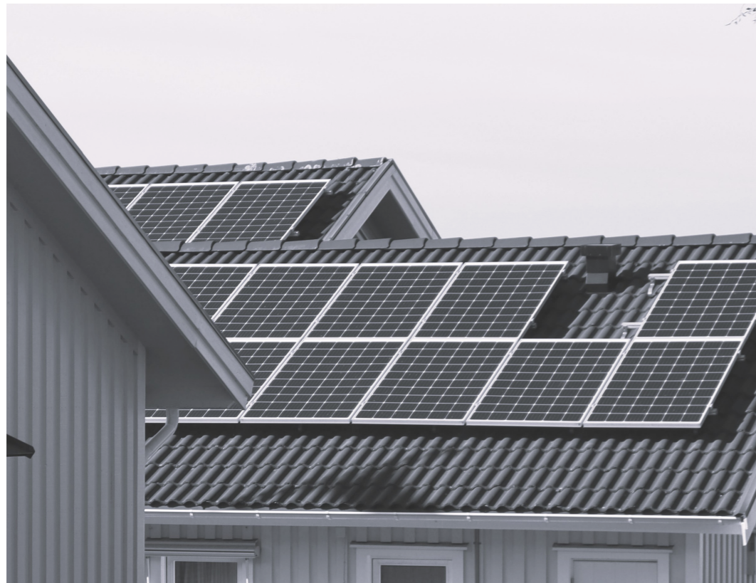
Photo 2. Solarpanels on existing roof in Ulebergshamn
