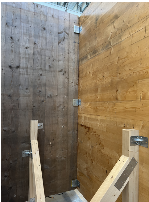
Figure 3.11: Christian Berners GePi100 mounted on the CLT-structure.
