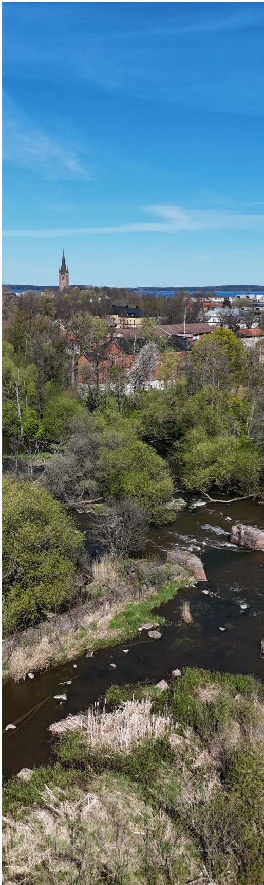
Image 22: Tidan's Kvillar, including existing foundations for a bridge
