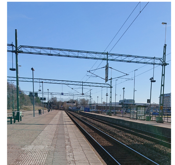
Trusses by train tracks. (Own photograph)
