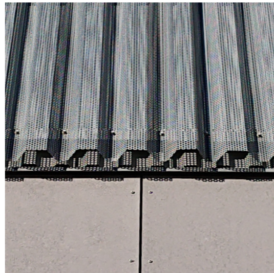
Perforated corrugated metal sheet. Own photograph from Innovatum
