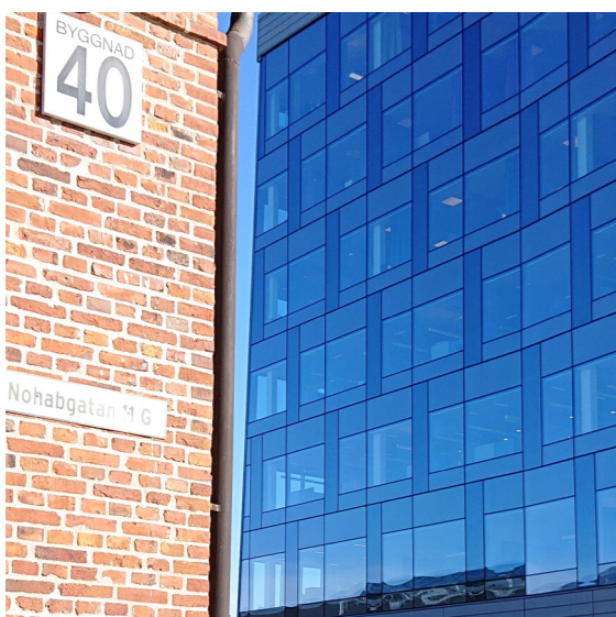
Glass facade relating to brick work. Own photograph from Innovatum.
