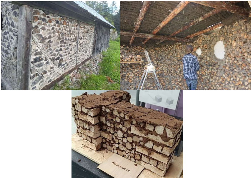
Figure 1.1: Examples of traditional scale cordwood buildings a) Barn in Hållnäs, Sweden, with walls built using a mix of cement binders and lime binders, the building is around 150 years old b) Cordwood house in Sweden built using a clay binder c) 1:5 scale model of cordwood wall using the lignin binder.
