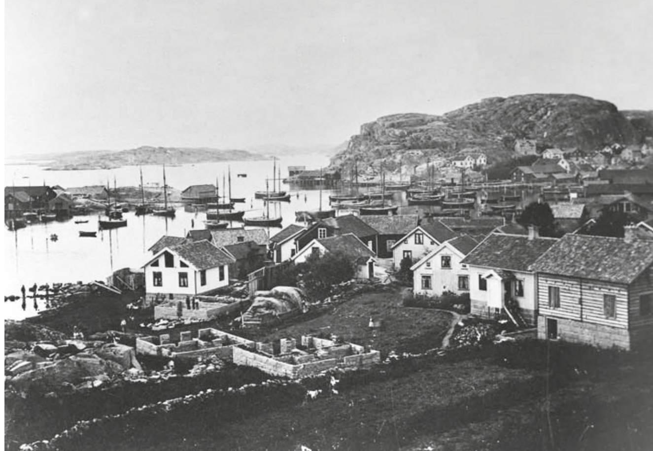
Photo 5-6: Historic pictures from Hunnebostrand and Udden, with prevalence of stone masonry
