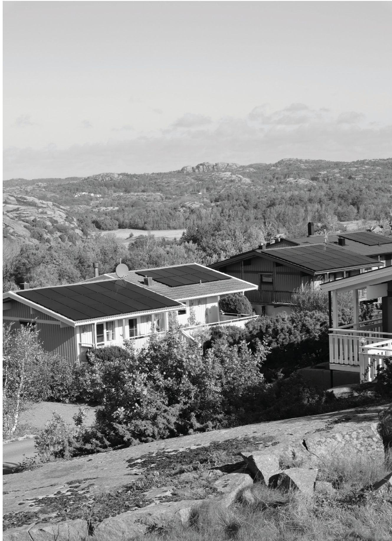
Photo 5: Solar panels added on numerous roof structures in Hunnebostrand, indicating a feasibility to integrate solar technology on the site
