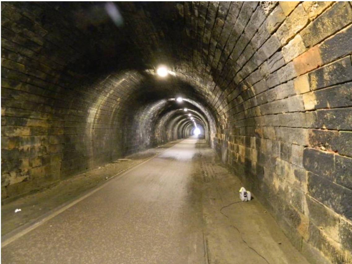
Figure A.16: The interior of the Innocent railway tunnel.
