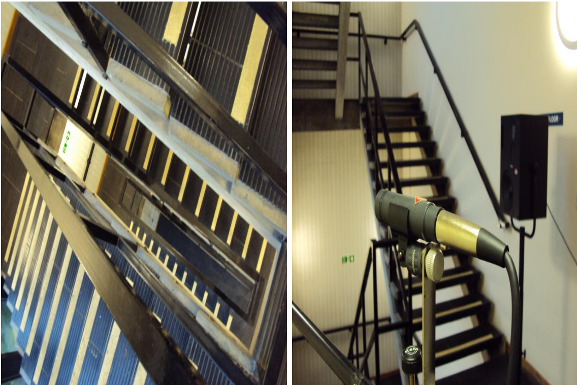
Figure A.8: The floor at which measurements were made at the Stairway (left). The floors below the measurement floor (right).
