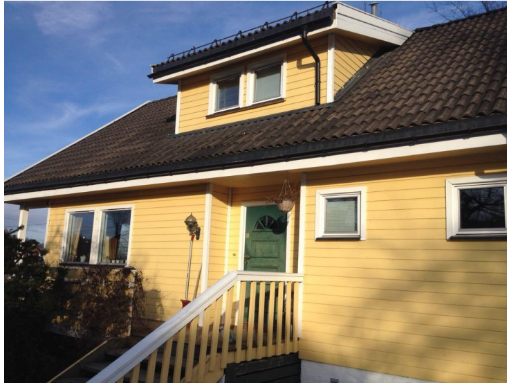
Figure 4-1: Picture of the facade of Jongsåsveien 31A taken by the homeowner.
