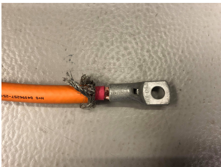
(e) Insert the conductor into the cable socket and press it. (f) Tape around the cutting area to separate conductor and shield.
