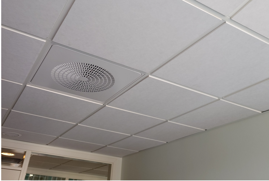
Figure 2.2: Picture showing a typical ceiling system installation with suspended porous ceiling absorbers.
