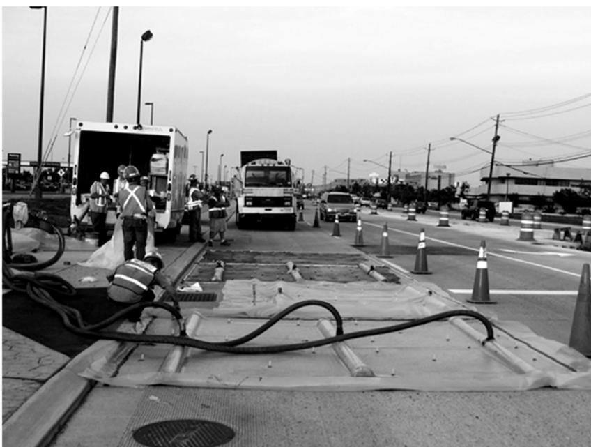
Figure 2.15 Vacuum treated concrete road slab (Balvac inc., 2007).
