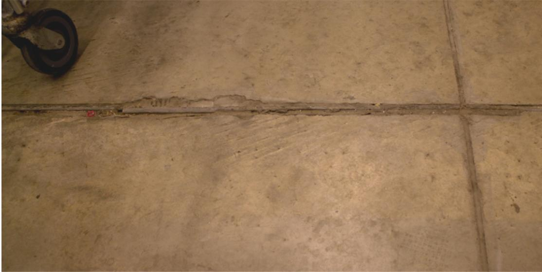
Figure 5.18 Example of problems with joint detailing for object 2.
