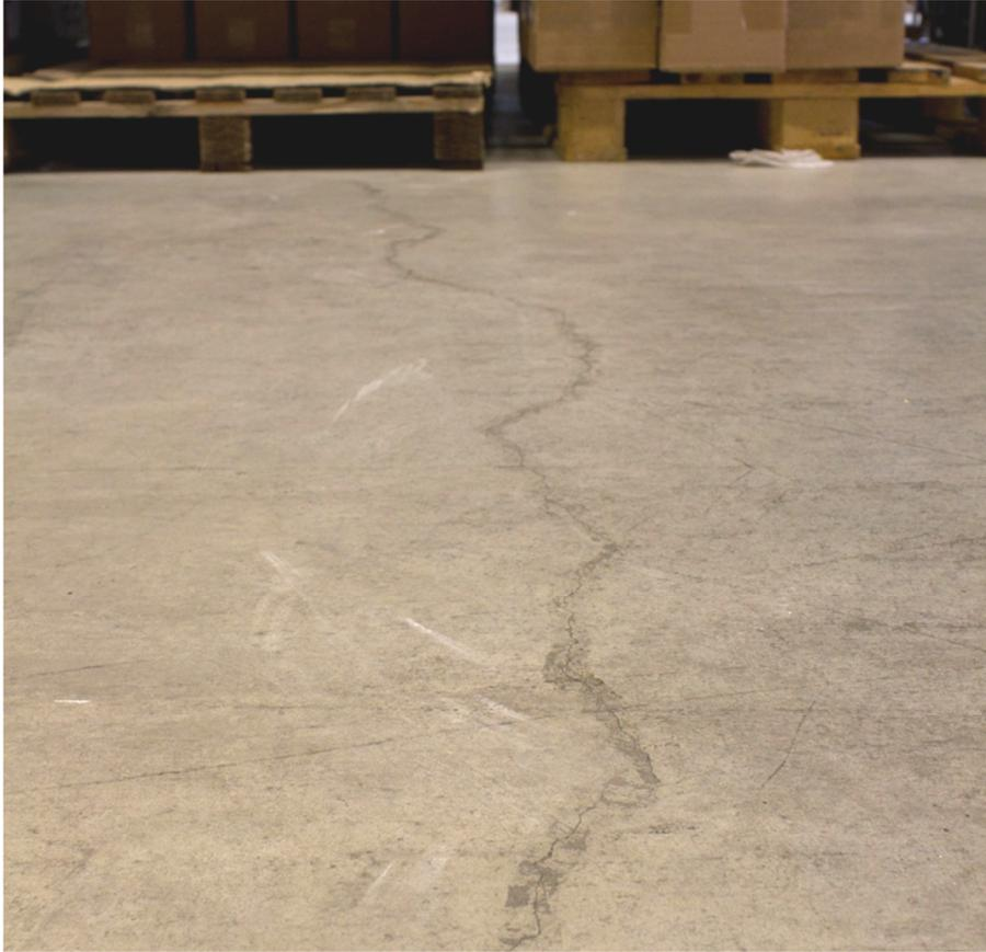
*Figure 5.32 Typical crack for object 4. The crack has been filled with an epoxy-based material.*
