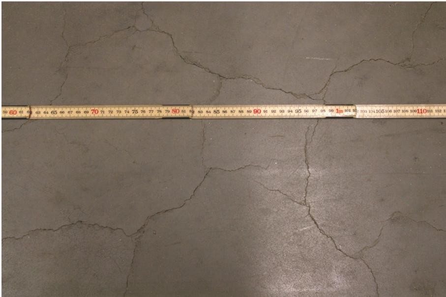
Figure 5.25 Typical crack pattern over pile for object 3.
