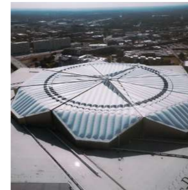
Figure 5. The retractable roof of Mercedes-Benz Stadium in Atlanta, USA (Byrom, 2023).
