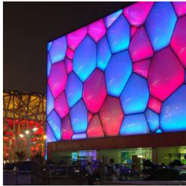
Figure 4. The ETFE clad facade of Water Cube in Beijing, China (Alerigi, 2008).
