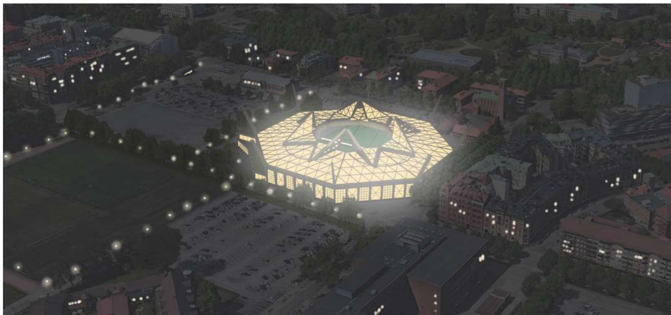
Figure 40. Aerial view during nighttime with open roof.
