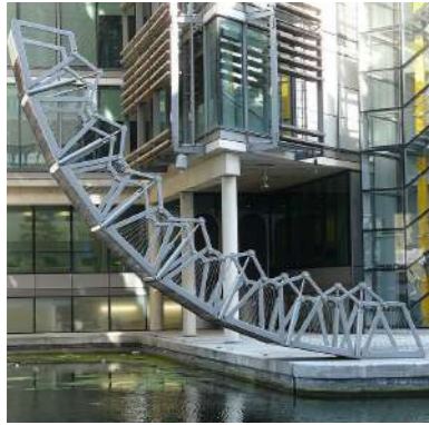
Figure 10. The Rolling Bridge (Pycock, 2013).
