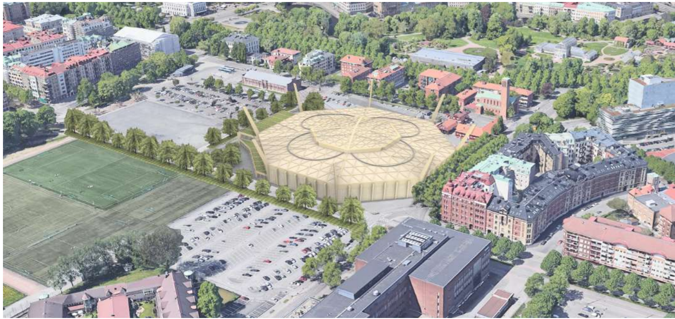
Figure 38. Aerial view during daytime with closed roof.
