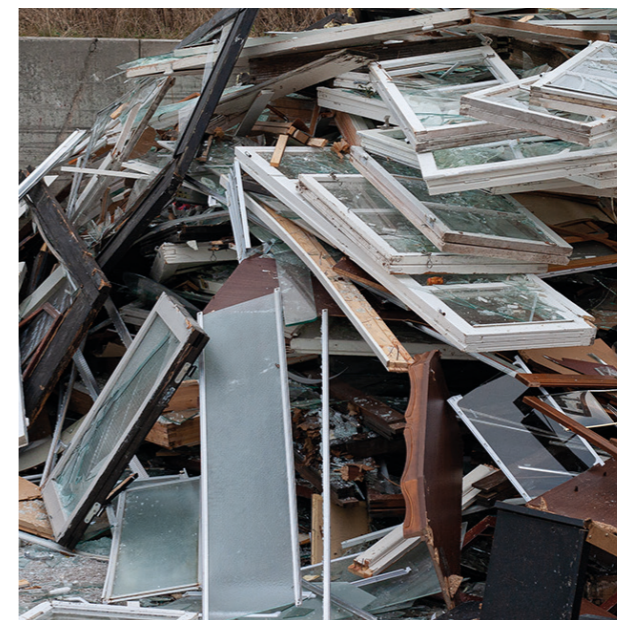
Discarded windows at a renovation Image: SSAM
