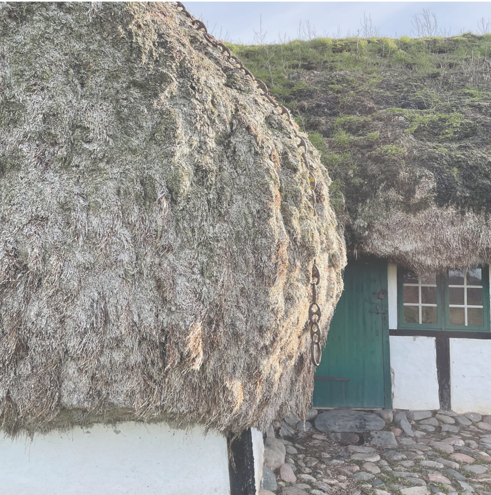
Farm building insulated with eelgrass from Bangsbo, Læsø
