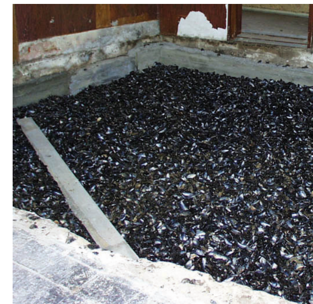
Mussel shell drainage in foundation Image: Bondegaard Rydbjerg
