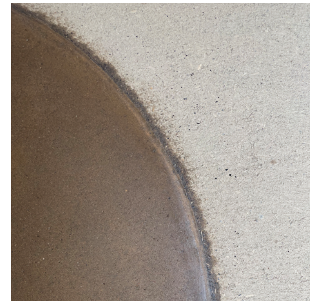
Waxed clay and clay wall surfaces
