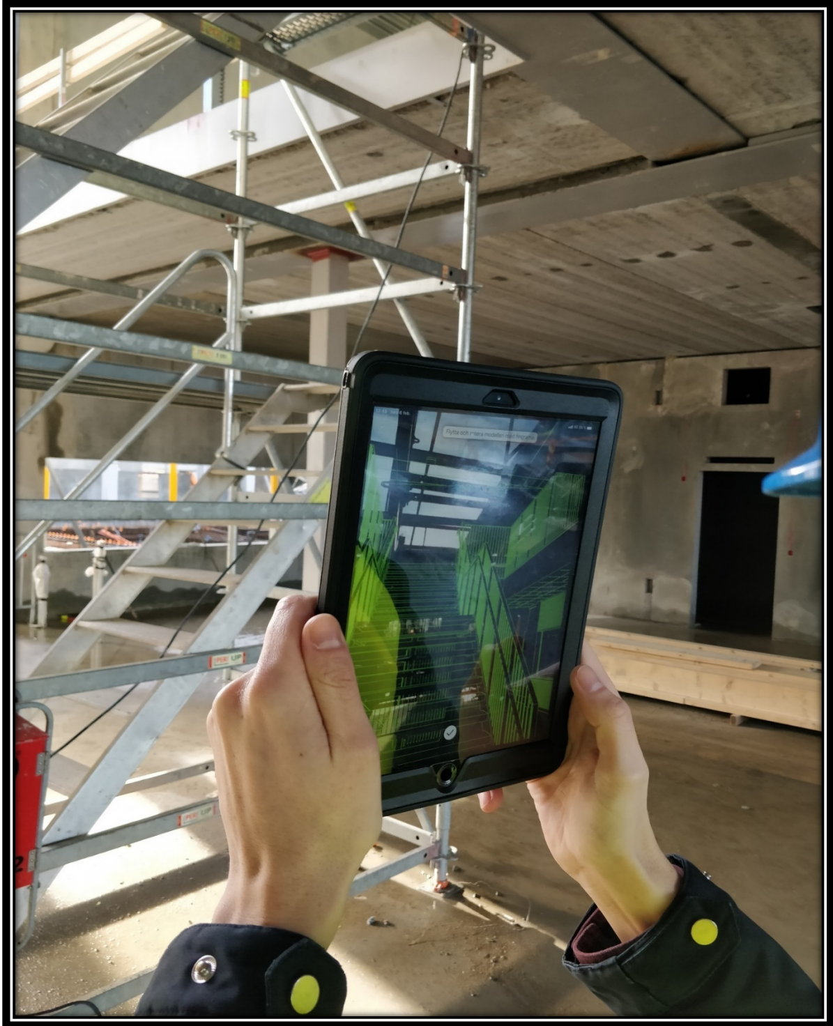
Figure 16 - AR through the Dalux TwinBIM application. Visualizing steel staircase in and open shaft.
