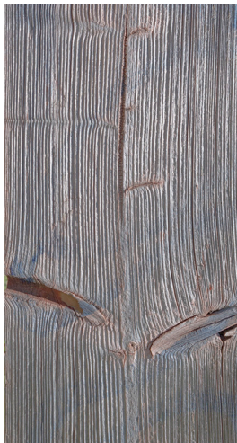
Post (silver damage) 180 x 150 mm x 1
