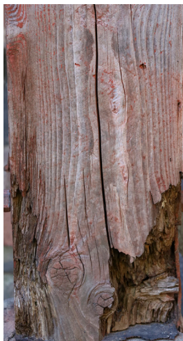
Post (rotten bottom) 200 x 180 mm x 1
