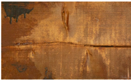
Rafter (in good condition) 220 x 180 mm x 6
