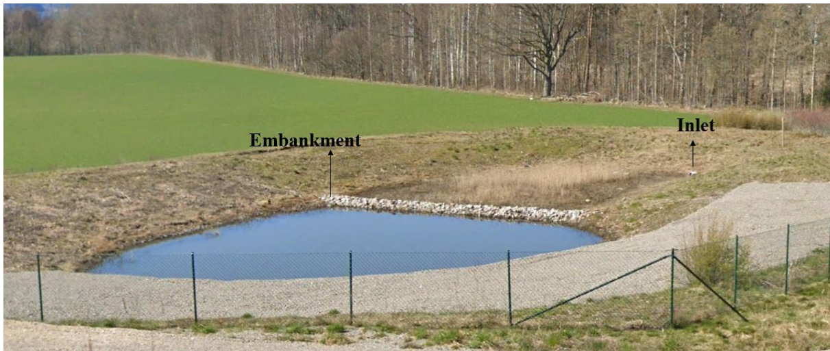
Figure T Pond with forebay to treat stormwater from E6 south Uddevalla bridge. Source: Street View.
