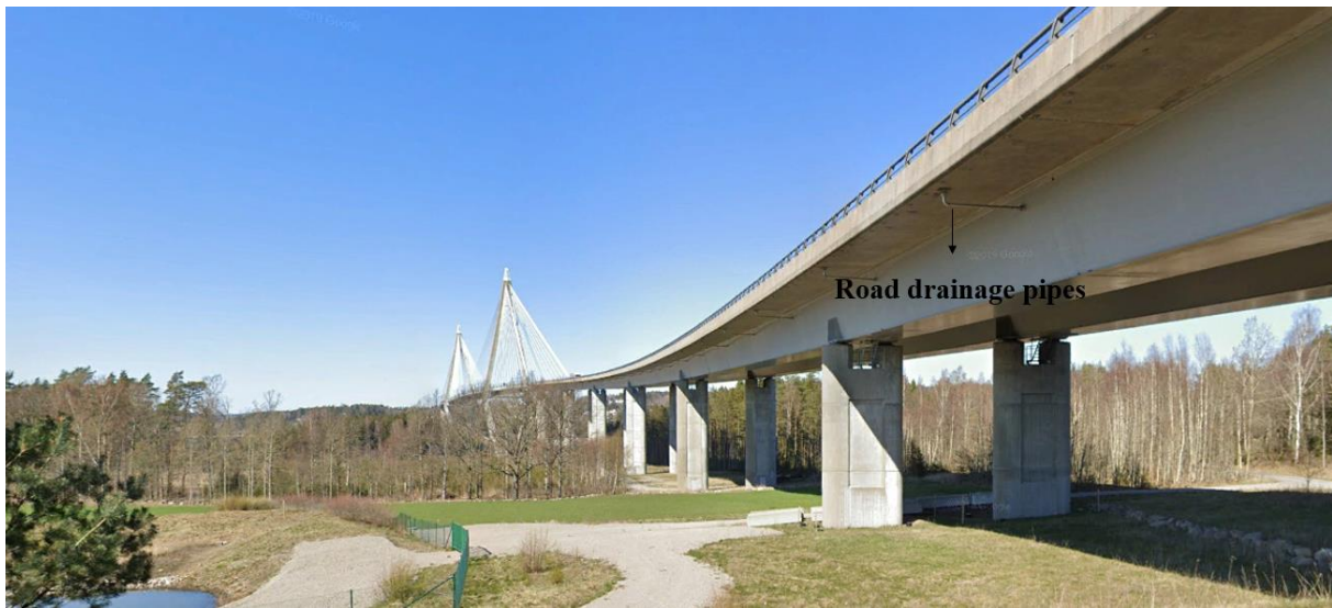
Figure V Road drainage pipes – E6 south Uddevalla Bridge. Source: Street View.
