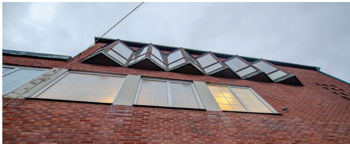
The slaughterhouse's borders and surroundings, January 2020
