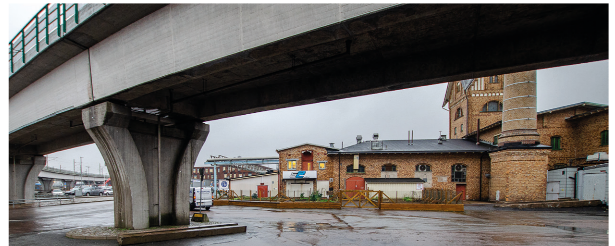
The slaughterhouse's borders and surroundings, January 2020
