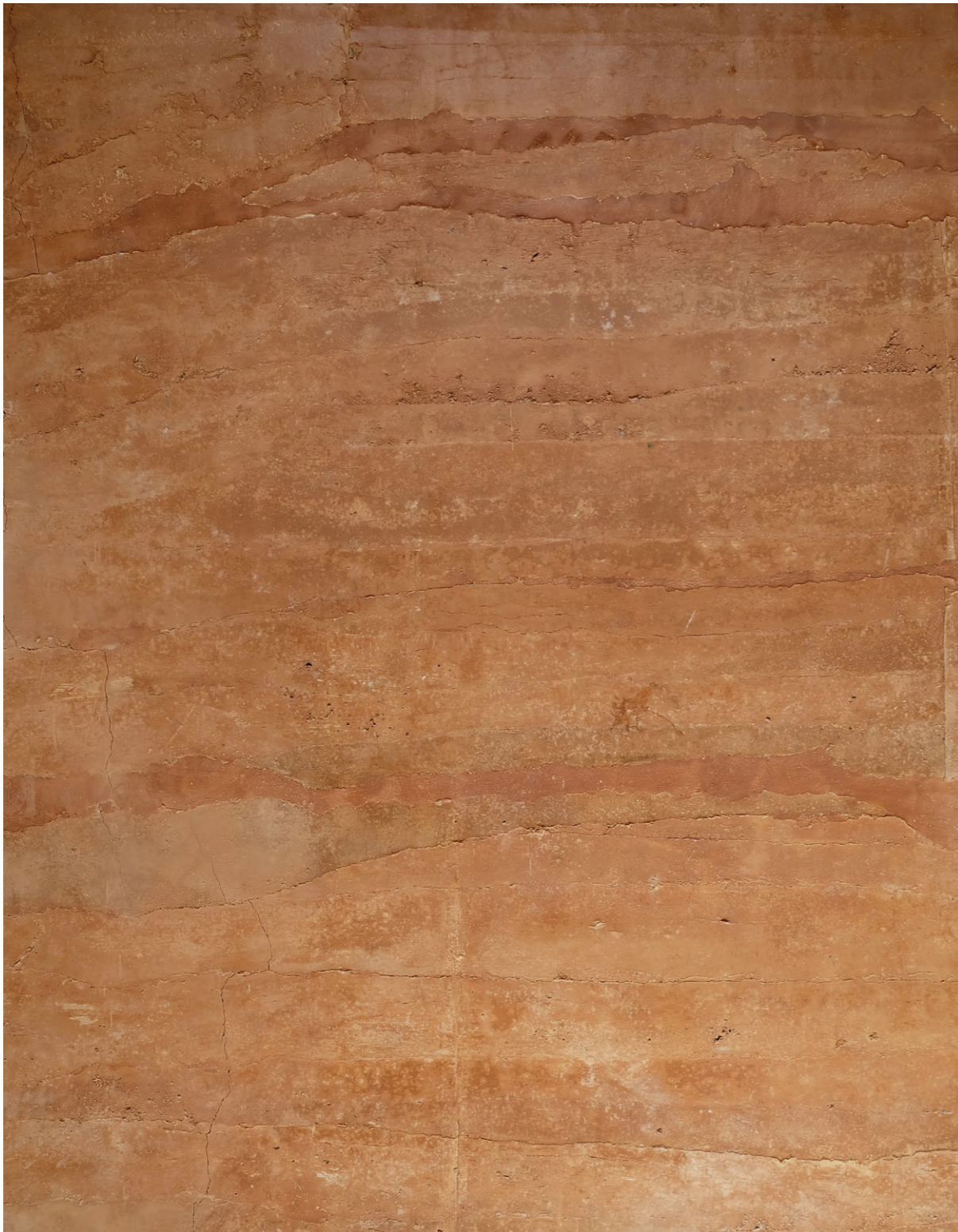
Figure 4. Red Rammed Earth Wall (Adobe Stock, n. d.).
