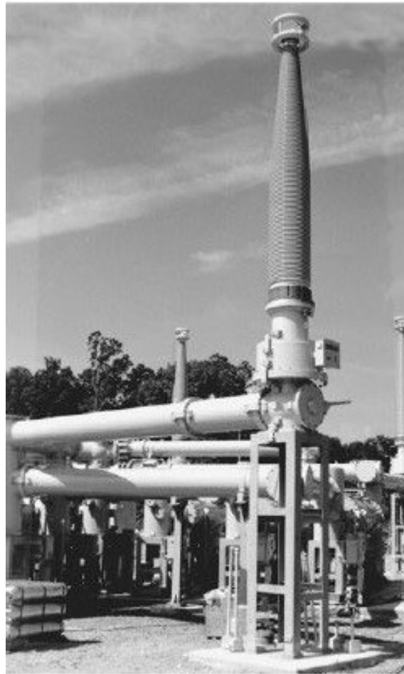
Figure 2.3: Air to SF 6 bushing [10]
