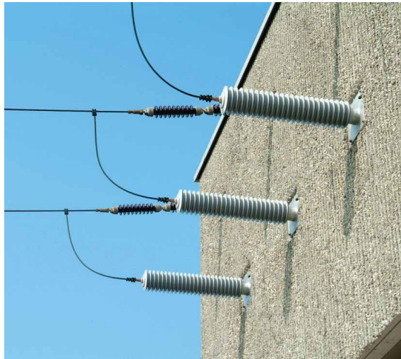
Figure 2.2: Air to air - Wall bushing [9]
