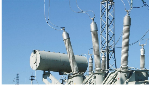
Figure 2.1: Air to oil - Transformer bushing [8]
